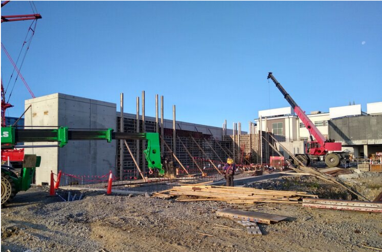
Hillsboro High School recently completed an $88 million full renovation and addition.
